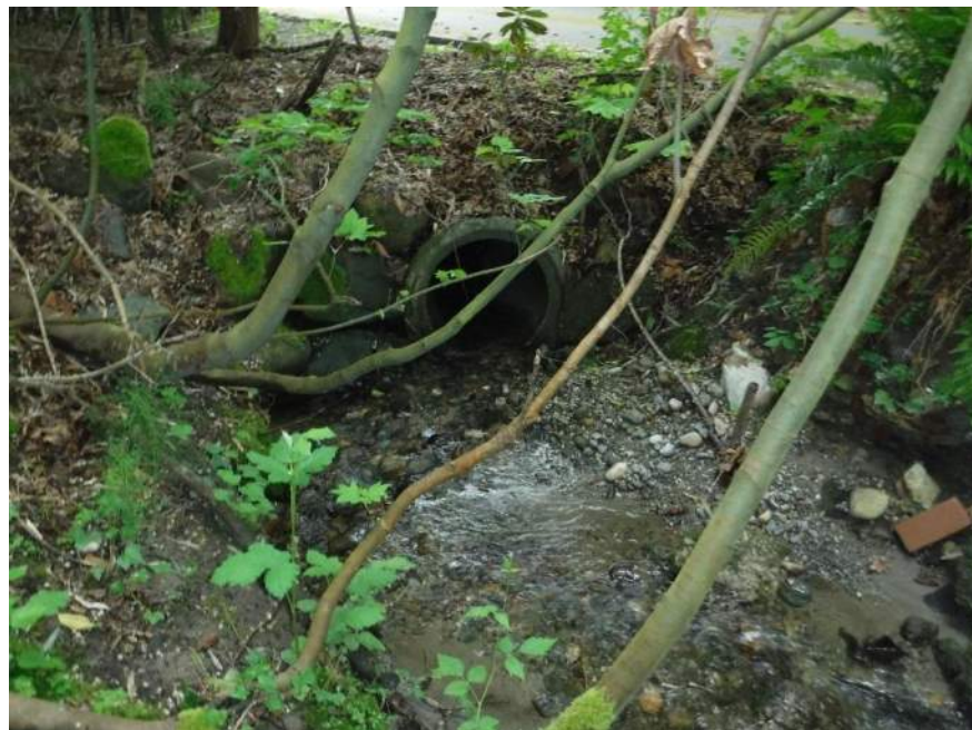
Image 8: Open channel flows inlet this 24" concrete culvert
